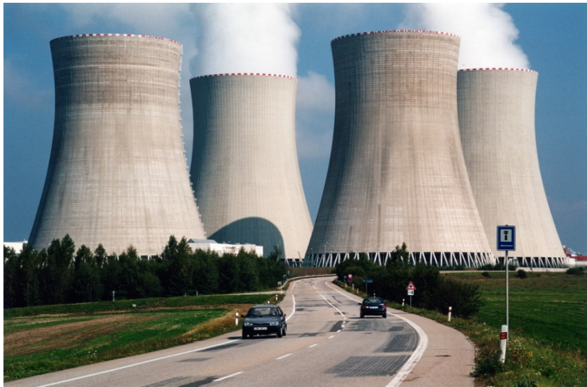
Nuclear Power Plant in Temelin
